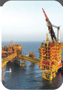
New Water Injection
